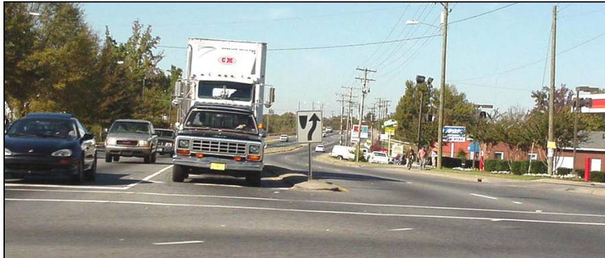
Crossing Harris Blvd. must be made safer for pedestrians.
