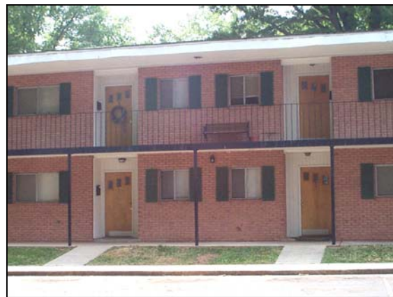
Design and development of multi-family housing is a key concern.
