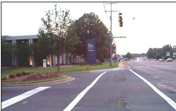
An example of a typical Eastside intersection without pedestrian improvements.
