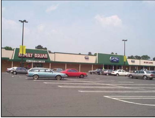
Retail disinvestment is occurring along Eastside Corridors.
